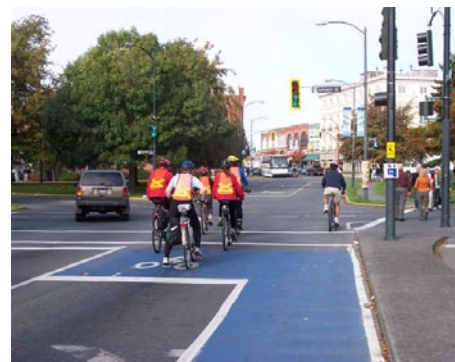
Above: Waiting in the Bike Box to cross Johnson St Bridge
